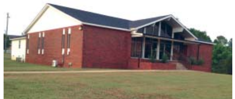
Operations Building for "House to House" in Jacksonville, Alabama
