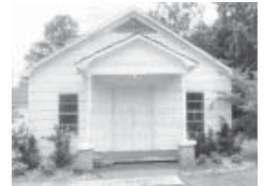
1956 Meeting Place Torn Down (Rotting lumber and termite damage)
